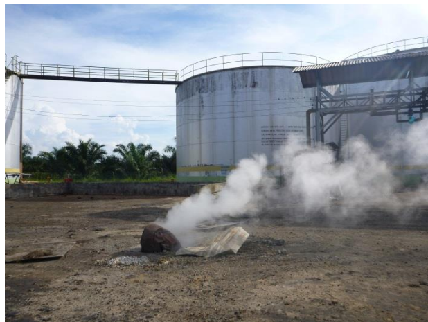
Figure 18: Leak pipes that cause hazard in the mill.
