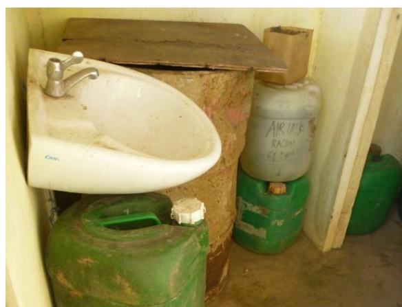
Figure 13: Herbicide containers used to store water in a workers' quarter.
