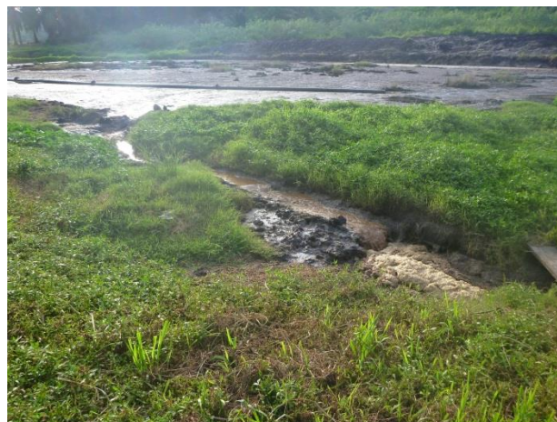
Figure 16: Evidence of overflow of effluent from one pond to another. Overflow might be contaminating the natural watercourse nearby.
