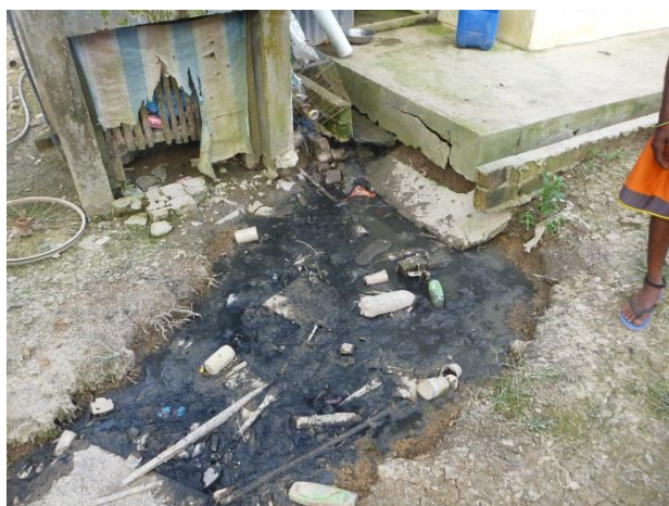
Figure 20: A workers' quarter with a dysfunctional sewage system and waste scattered around.
